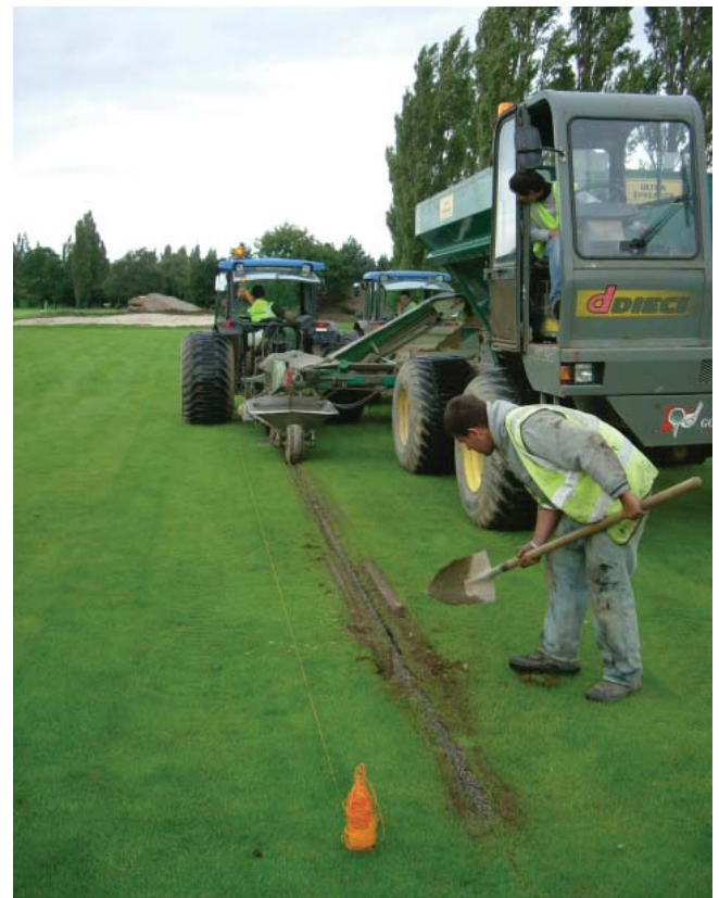
DRAINAGE CONSTRUCTION DEMONSTRATION BY SOL GOLF CONTACTORS
